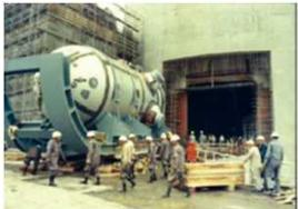
June 1969 Unit 1 Installation of reactor vessel
