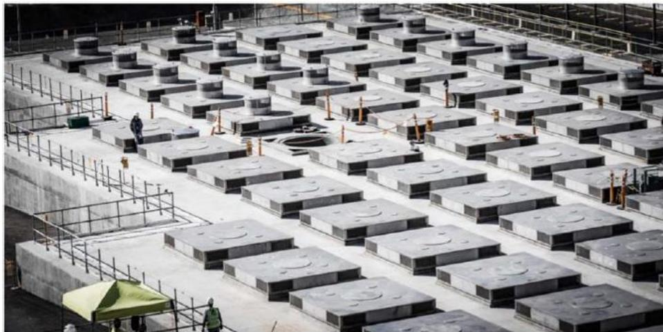
Figure 3 - The Holtec UMAX storage system at SONGS
