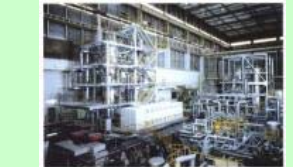
Helium Engineering Demonstration Loop (HENDEL)
