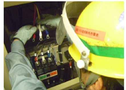
(直流き電盤内NFB2次側へ接続)
