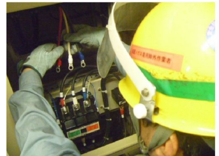
(直流き電盤内NFB2次側へ接続)
