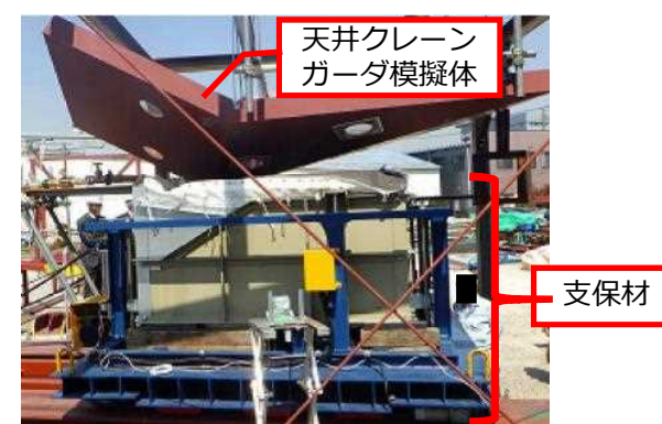
③支保材自走(完了)
